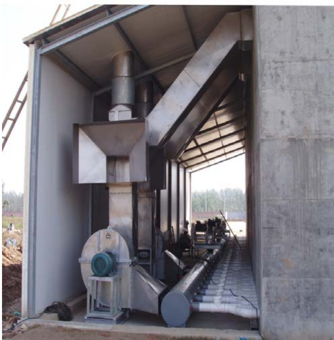
Photograph of 300 tonne phase II tunnel with no fans and dampers into the same plenum
